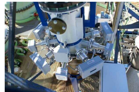
Laser gas monitor
