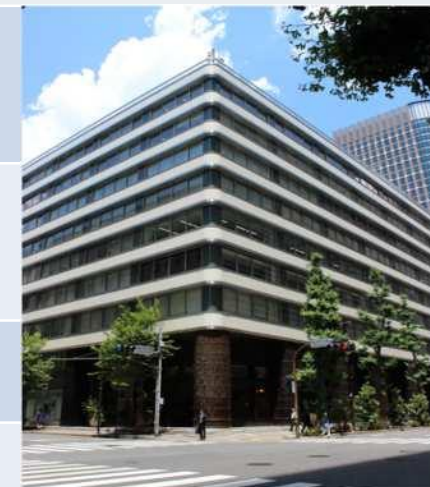
Head office: Shin-Tokyo Bldg., Marunouchi
